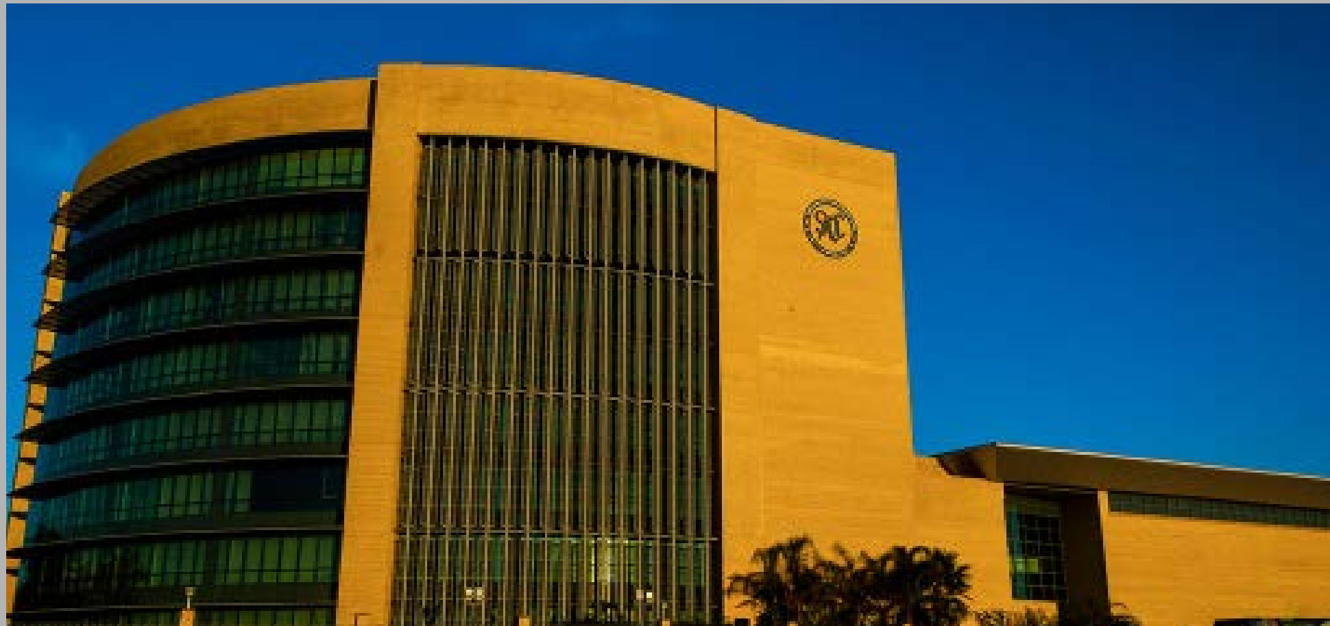
SADC headquarters. Pic: www.area.co.bw
